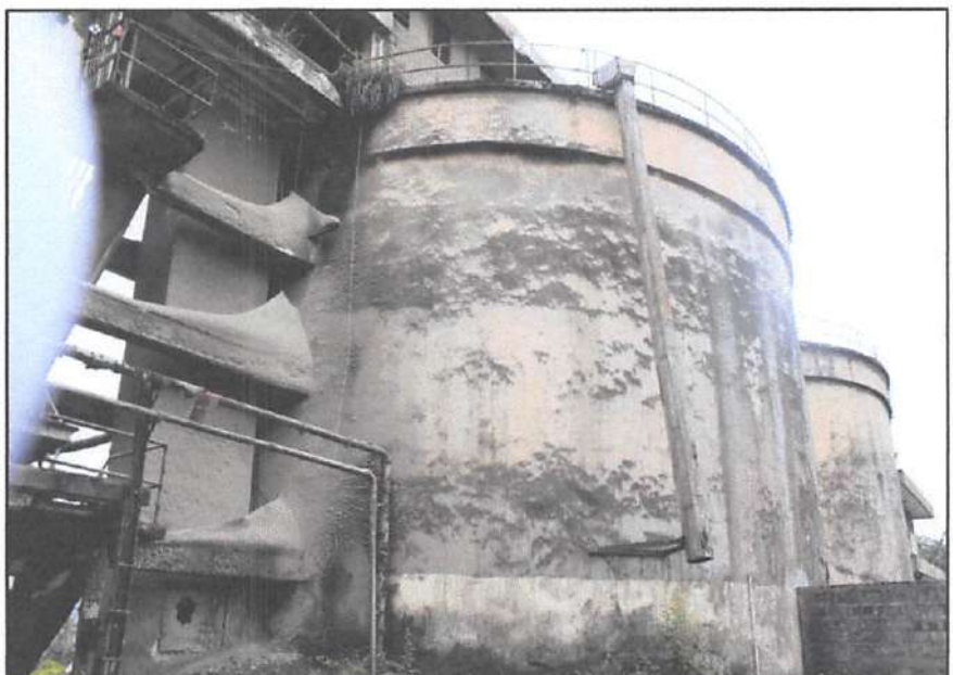
Foto Silo Semen B ( Cement Silo B ) Tampak Samping
