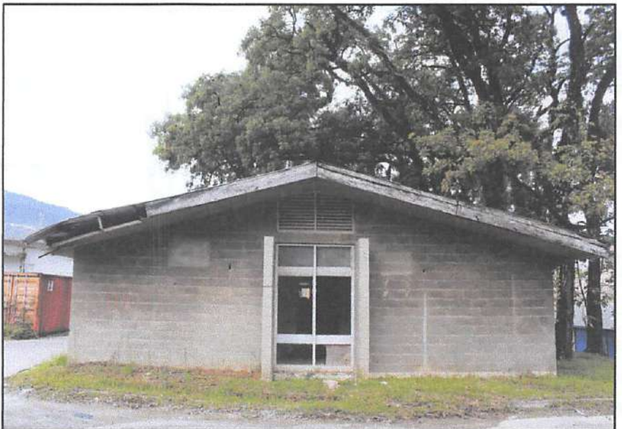
Foto Kantor Penelitian dan Pengembangan ( Research & Development Office ) Tampak Samping
