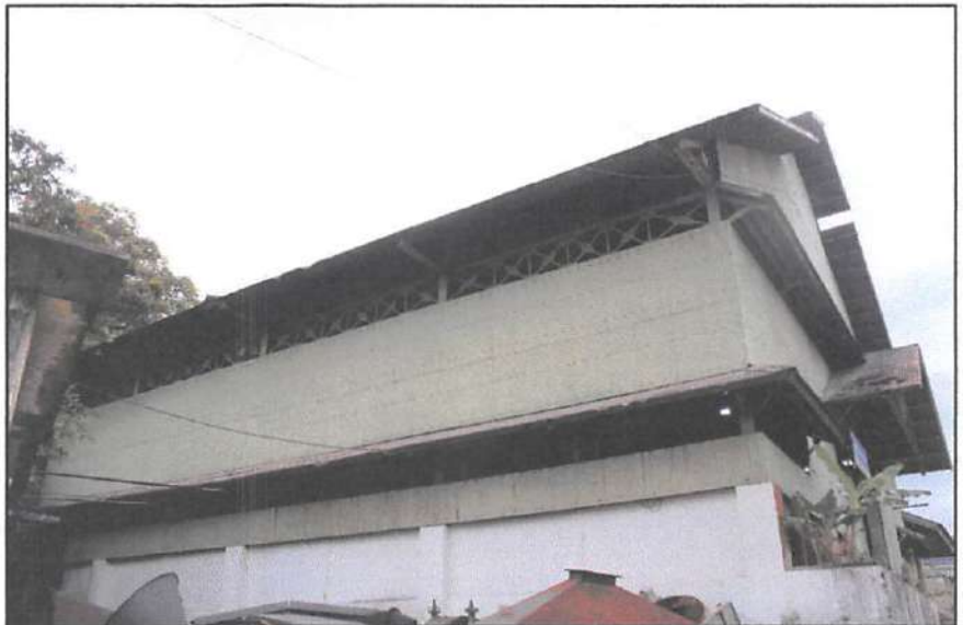
Foto Bengkel Listrik ( Electrical Workshop ) Tampak Samping Kiri
