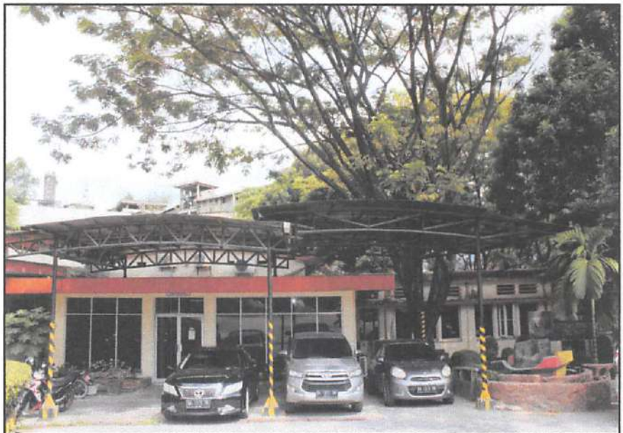
Foto Laboratorium 25 ( Laboratory 25 ) Tampak Depan
