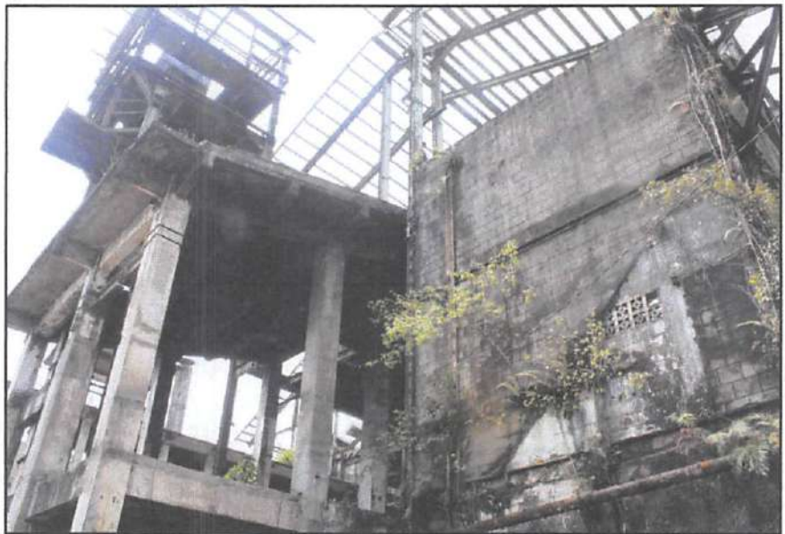
Foto Pabrik Batu Bara ( Coal Mill ) Tampak Samping
