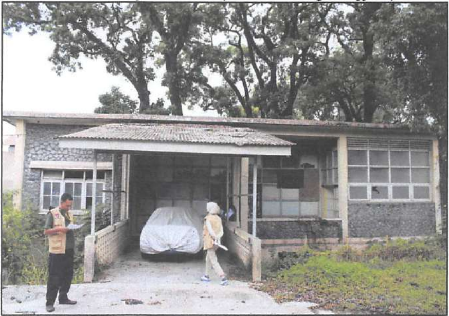
Foto Kantor Manajer Pabrik ( Plant Manager Office ) Tampak Depan
