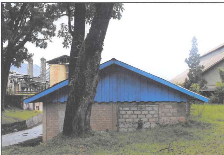
Foto Gudang 30 ( Storage 30 ) Tampak Samping Kanan
