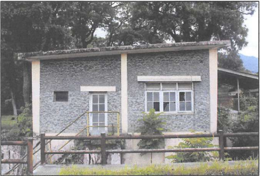
Foto Kantor Manajer Pabrik ( Plant Manager Office ) Tampak Samping Kiri
