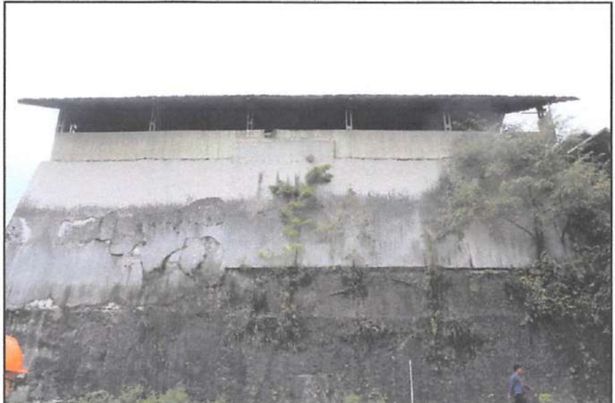
Foto Silo Batu Bara ( Coal Silo ) Tampak Samping
