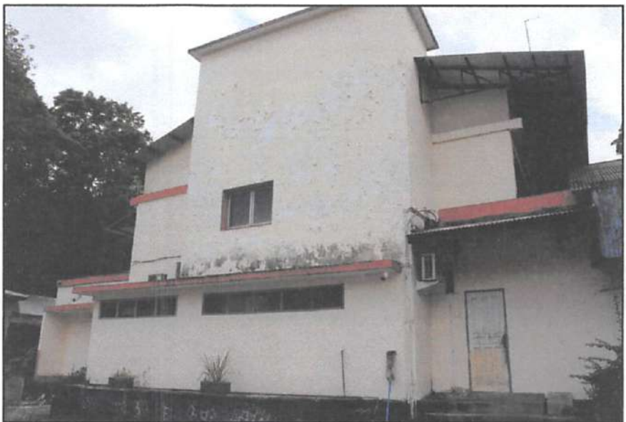
Foto Gudang 26 ( Storage 26 ) Tampak Samping Belakang
